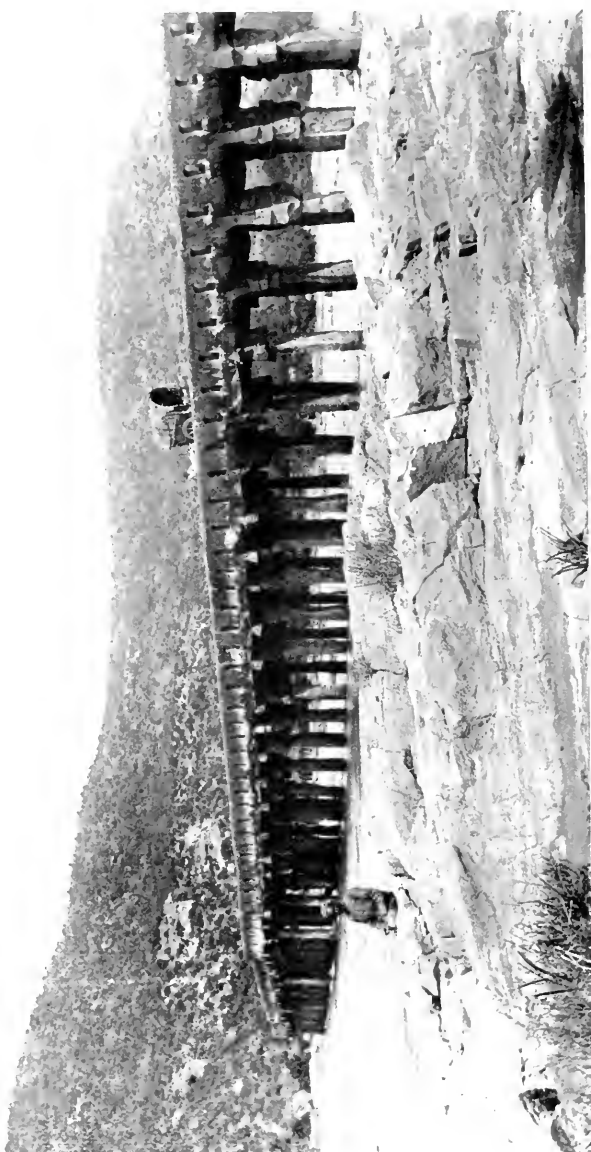
Fig. 27. Bridge made of slabs of gneiss split by fire.
